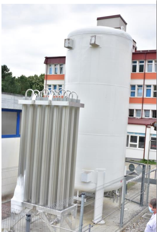
Cryo-tanku 10 ton, SP Pejë
